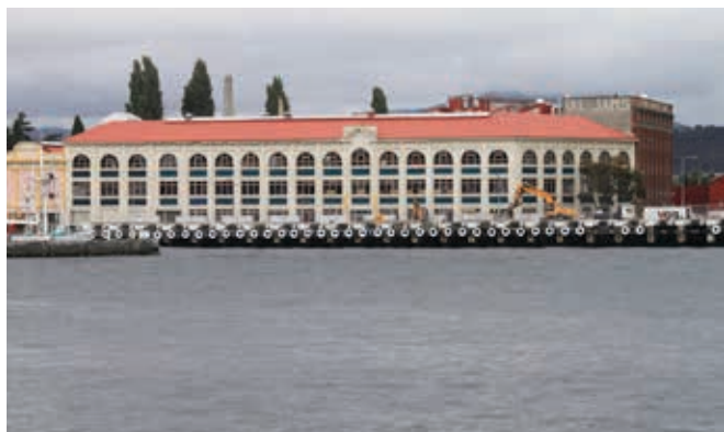
View to Jam Factory (UTAS School of Art) early 2015 after Shed 1 was demolished Photo: Rex Cox
