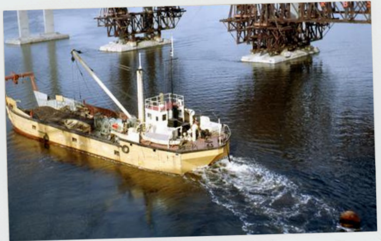
Barge B4 at the Tasman Bridge site, August 1964 (photo: Rex Cox)
